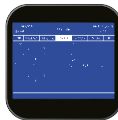
UPS Kabin Kontrol Paneli
